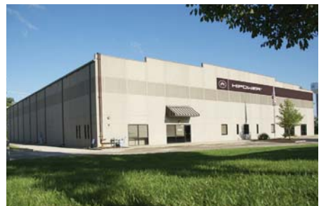
HIMOINSA POWER SYSTEMS INC.
